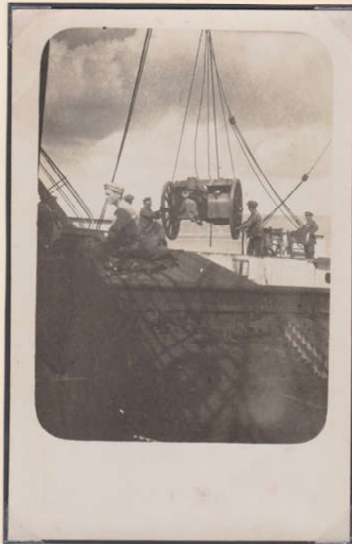
Post card showing field guns being off loaded from a ship, possibly at Salonika. The labourers appear to be Central Power P.O.W. by their uniforms supervised by a British officer.
