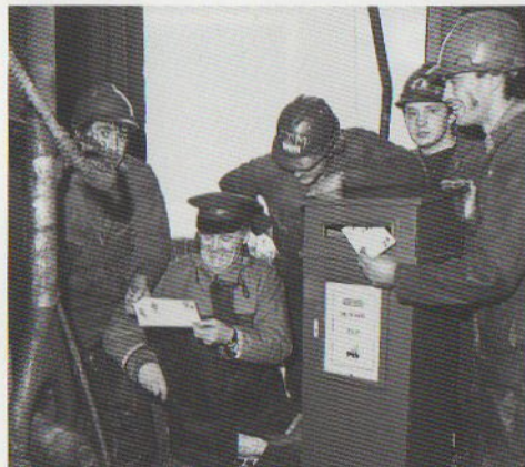
A temporary posting box was established on the Conoco Hutton oil platform on 14 January 1986 when the Industry Year stamps were issued. The 17p stamp featured a North Sea platform.
