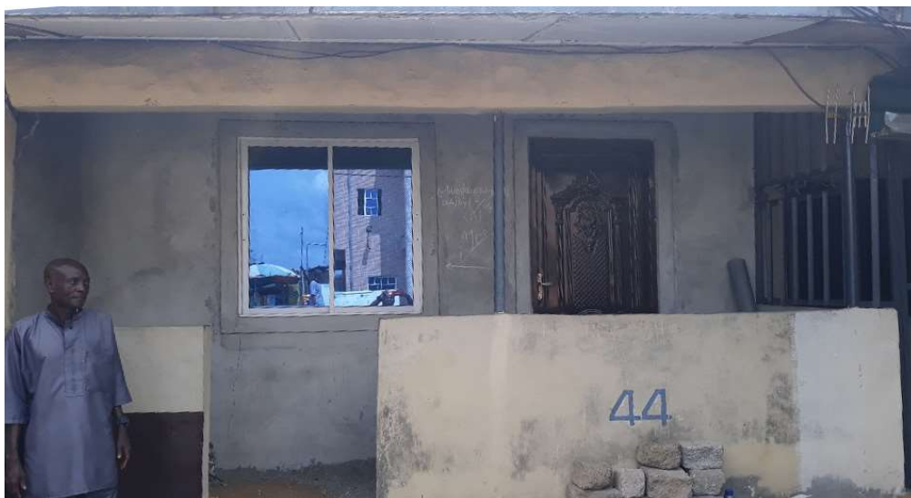
Efut postal agency building at 44 Edgerley Rd, Calabar
