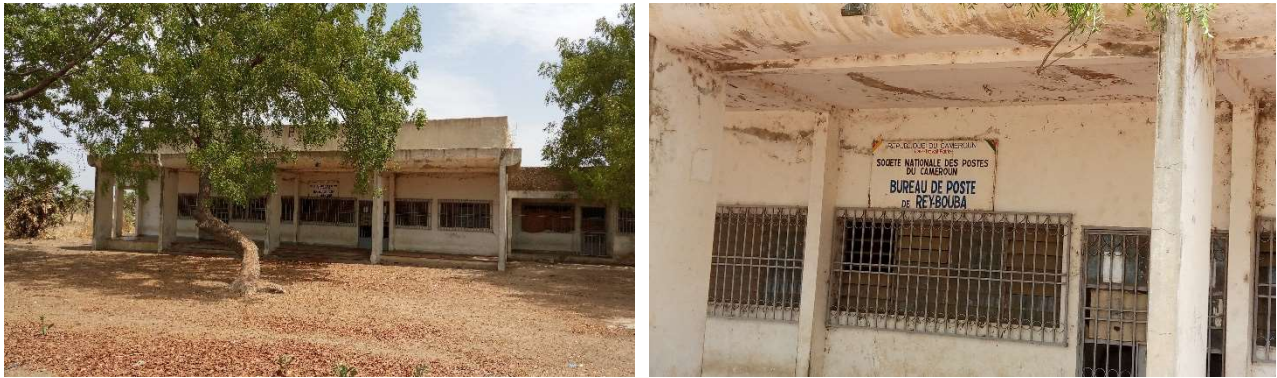
Figure 25. The old Rey Bouba post office temporarily closed, April 2018. Photo – Marc Parren.
