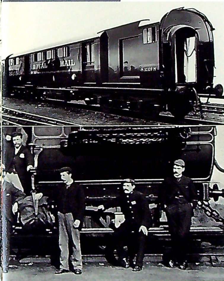
Above: Staff on the Midland TPO
