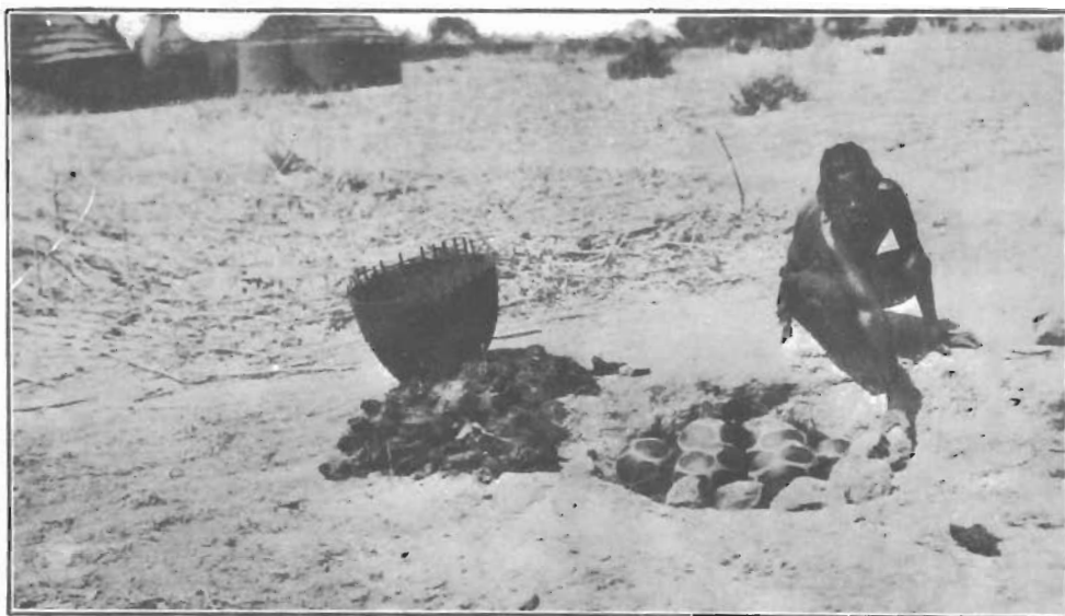
FIG. 2.—POTS STACKED IN KILN.
