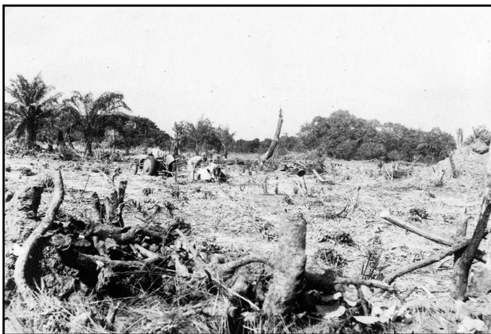
Here is what Jim Adams had to face at the runway site for Benson. You can barely make out the tractor, but this was the runway centre line.
