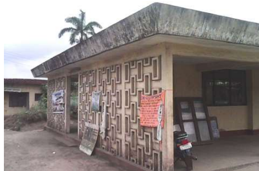
Eket PO, which is to be demolished for road widening
