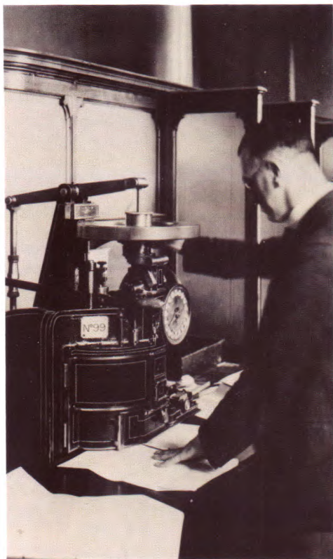
Somerset House, Room 28. Behind the counter in a public stamping room (with a stamping machine of 1913). Principal Stamper at a high duty Recording Press. (Courtesy Inland Revenue)
