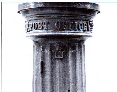
6. Ridge on main column stopping tablet from being removed
