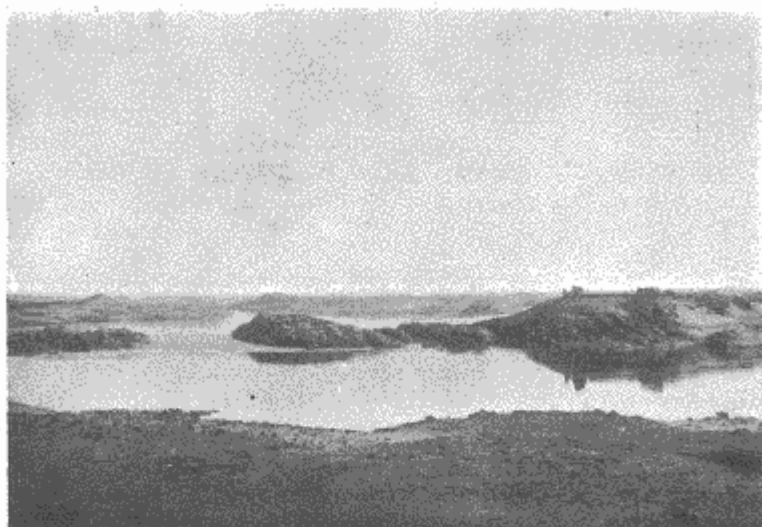
SEMNA CATARACT AND THE EAST FORT, LOOKING NORTH, FEBRUARY, 1924.
