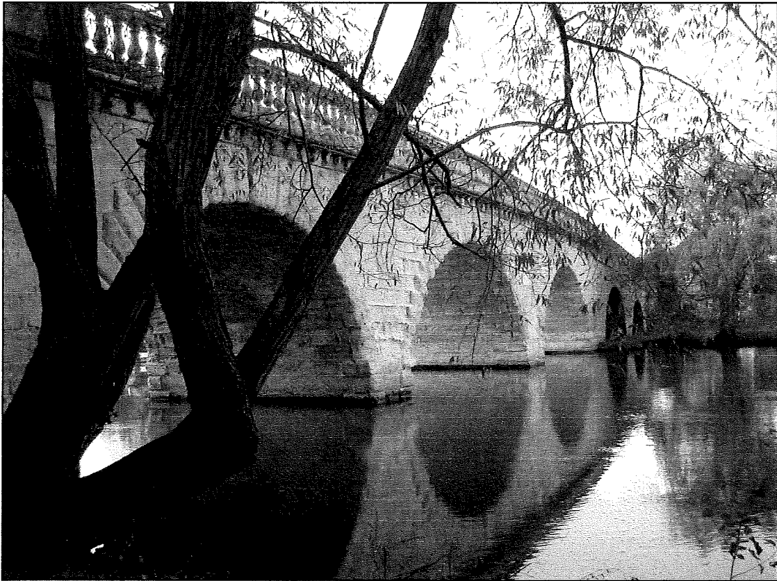
Swinford Bridge in October 2008
